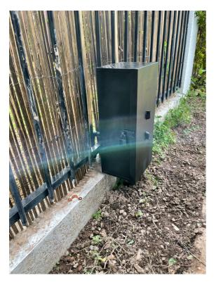
The box houses the on off tap and the 9 volt battery controller unit. Inside the box is also the tool for adjusting sprinkler flow and radius. The key to open the box is attached underneath the bottom of the box with a magnet
