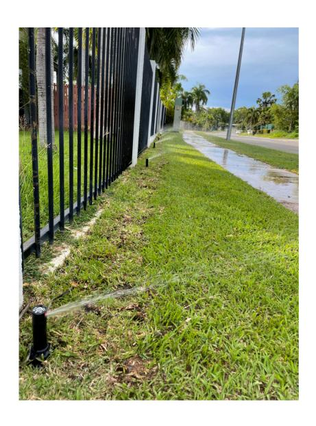
We dug up and replaced the 25mm supply pipe and installed 7 Rain K1 gear driven sprinklers. 4 meters apart. The sprinklers overlap and reach the roadside.
