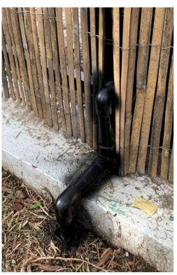
Used unit 10's garden tap already installed next to the water meter. With very good pressure. Joined on to the existing tap and went back down underground the front fence were it comes up and into a service box mounted on the fence. (New works all in black- The black stop cock controls pressure. Strapped off in set position)
